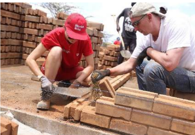
Production of Interlocking Stabilized Soil Blocks (ISSB) on site during construction
